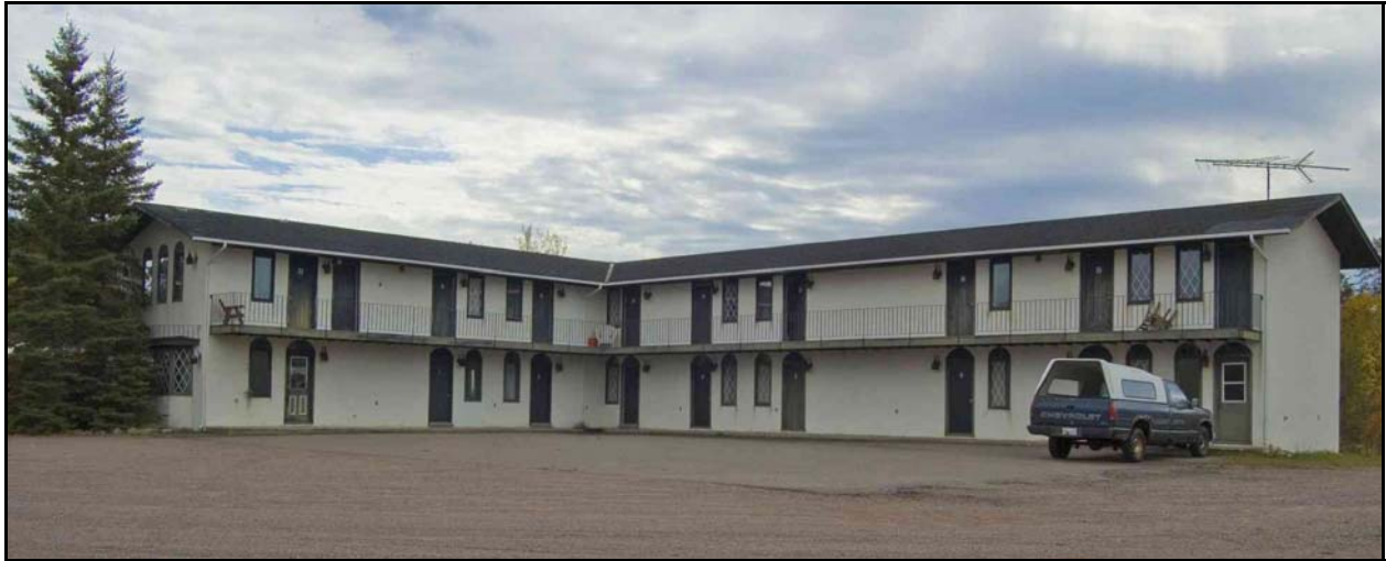
Front View of the Fallen Rock Motel
