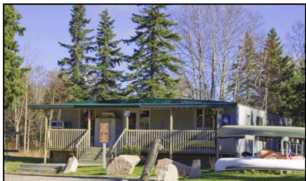
Campground Office – Visible from Highway
