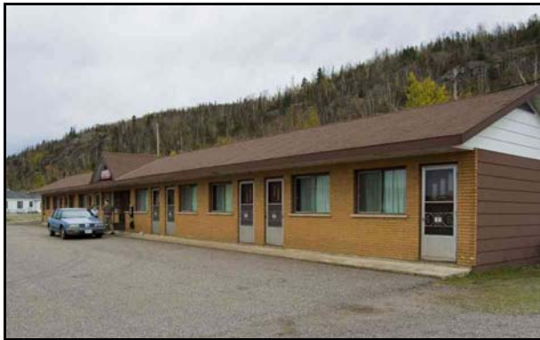
View from the Highway of the Sunset Motel
